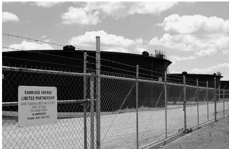
The Enbridge crude oil tank farm in Cushing, Oklahoma, has a maximum storage capacity of 20,060,000 barrels.
