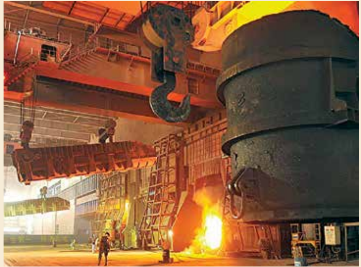
Converter, hot rolling department, main plant of HBIS Tangsteel, Tangshan, Hebei, China.
